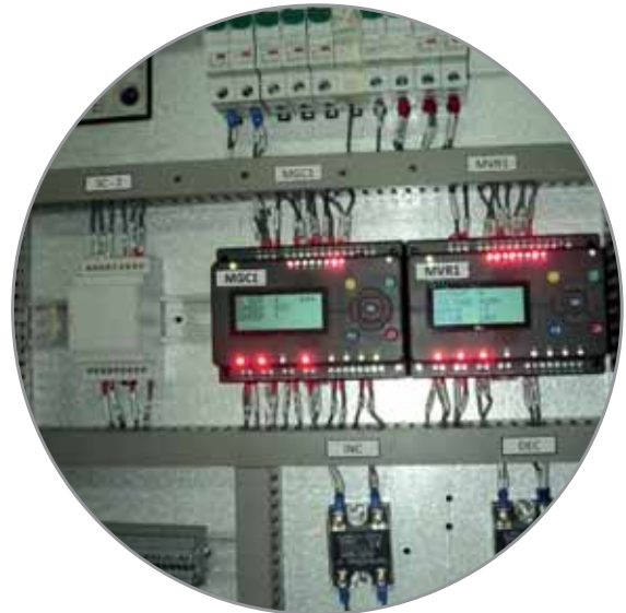
MIACs used to control a mid scale hydroelectric power station in Sri Lanka.
